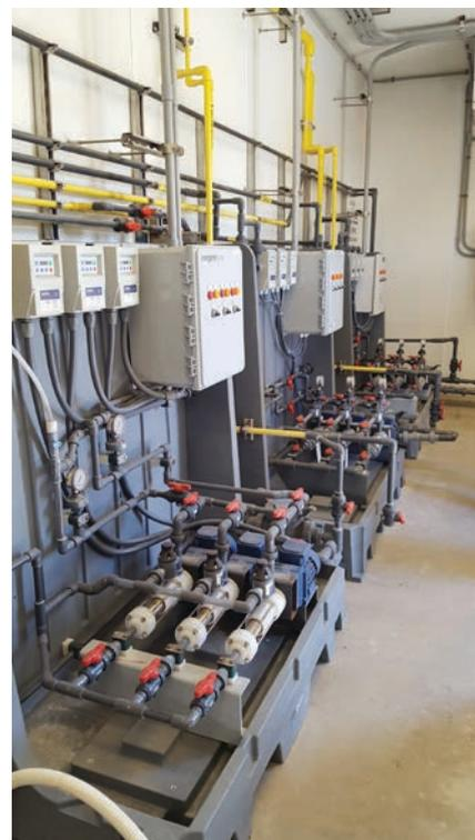
**The series of PC chemical metering pump systems provide accurate metering of sodium hypochlorite (bleach) during treatment to produce drinking water. SEEPEX**
