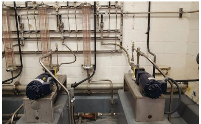
**PC metering pumps used sodium hydroxide (caustic) at the City of West Palm Beach Water Treatment Plant. SEEPEX**
