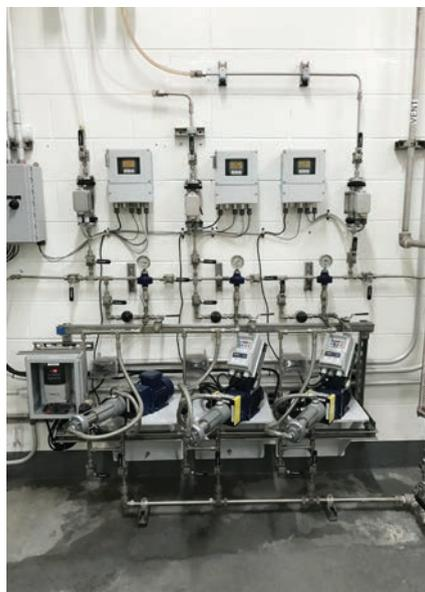
**PC metering pumps with variable frequency drives provide operators with integrated and easy-to-use control of the pumps. SEEPEX**
