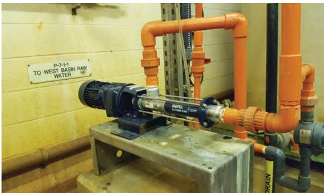
**SEEPEX PC metering pump used to dose ferric compounds at the Florida drinking water facility. SEEPEX**
