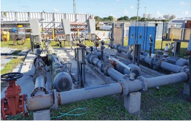
PC sludge pumps used feeding sludge to a belt press. SEEPEX
